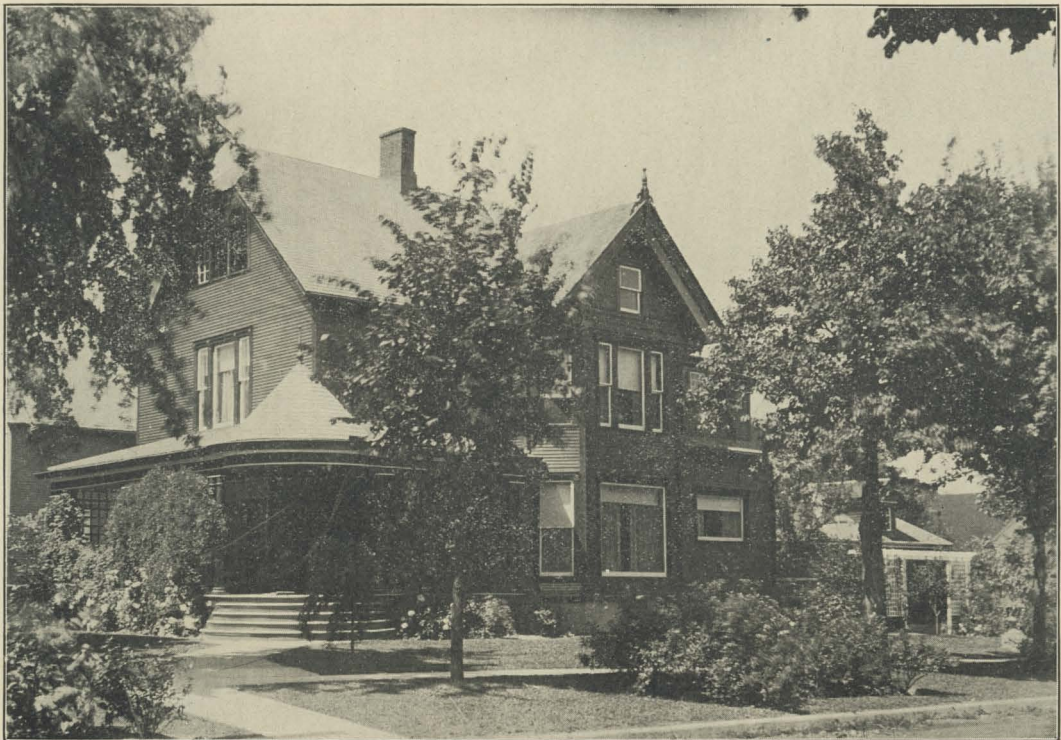
Residence of John W. Sieb
