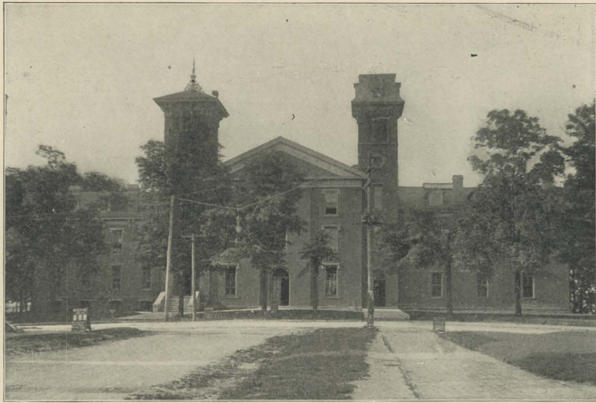
Old College Building as it Now Appears
