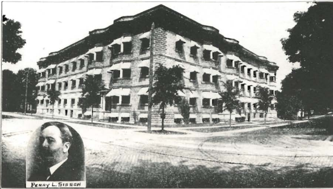
Pioneer Apartment Building, erected on the old Marks corner in 1908 by Perry L. Sisson, is still in use today.
