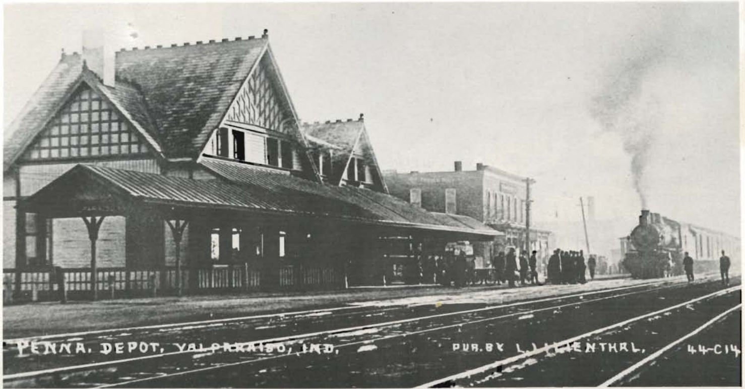
Pennsylvania Railroad Station - Early 20th Century
