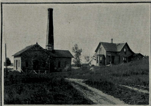
Water Works - Pumping Station.
