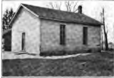
One-room Frame Building, Porter County. Erected about 1862.
