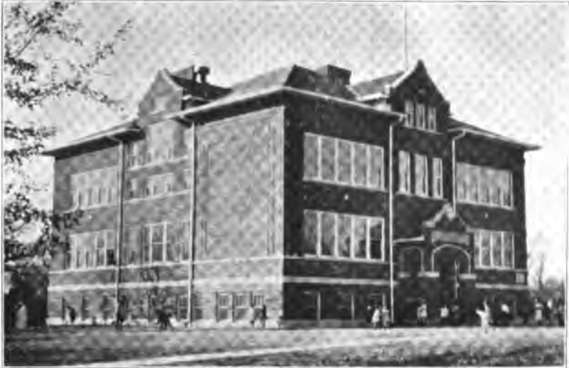
Modern Township Consolidated School, Porter County.
