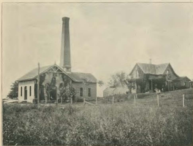
WATER WORKS AND GROUNDS, VALPARAISO, IND.
