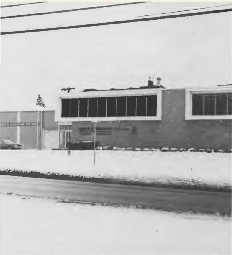
DAVID E. McDANIEL COMPANY, INC. are specialists in the installation of automatic fire protection. Located at 1055 W. Joliet Rd., they suggest that you don't gamble with fire because the odds are against you.
